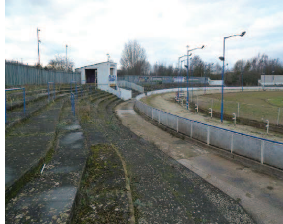
Fig 4: The concrete western terraces (built c 1939) are in many ways exemplary of their time both in their design and materiality (i.e. form). Their location in quite close proximity to the dog tracks catered to the 'modern desires' of their audiences who increasingly sought more heightened sensorial stimulation through greater contact with the 'main action'. Their curving design following the general line of the track enable spectators to view the unfolding of a race from start to finish without the need for binoculars as was often the case with other sports such as horse racing. Their material construction – consisting primarily of large expanses of moulded concrete - embody the modernist movement's preoccupation with ephemeral as well as catering to the need for expedience that was generally necessitated in the construction of pleasure buildings.
